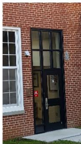
SMS, BHS Install canopy at main entrance
