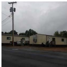
CES Replace Mobile units with modular units
