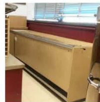
SMS Replace through-wall heating units
