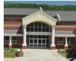
EMHS handicap auto door openers at main entrance
