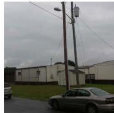
CPS Replace Mobile units with modular units
