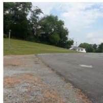
CES Additional Asphalt for parking
