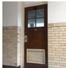
SMS Replace classroom, restroom, and other interior doors
