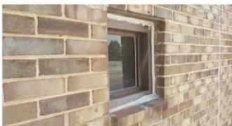
CHS Replace Library Windows CT
