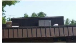
CPS HVAC Unit replacements
