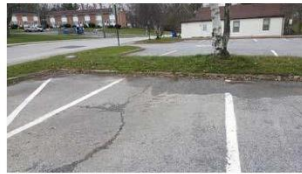
HAE Overlay/re-pave asphalt parking lots and drives, rebuild curbs, Increase number of marked and paved parking spots. Replace sidewalks
