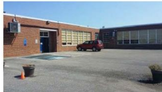
Technology Building - Replace windows Montgomery Central Replace windows- lower building
