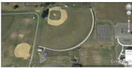
AHS baseball field dugout improvements
