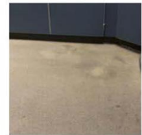
EMHS Replace Main office flooring
