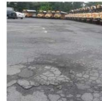
Cambria complex & Technology Center Pave/overlay asphalt parking lots
