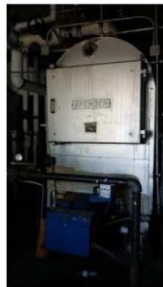
CPS Install new boiler - CT
