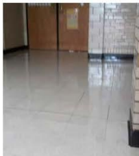
SMS Replace floor tile
