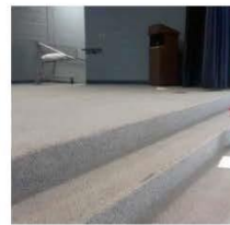
KES Replace Stage Flooring
