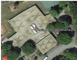
HAE HVAC Units Replacement
