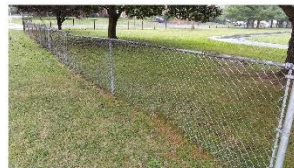
MBE & GLE Replace Fence at front
