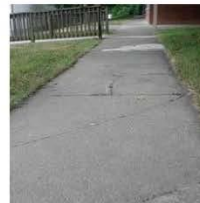
CES Replace deteriorated sidewalks
